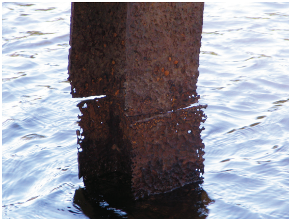
Steel H-pile corroded completely through (left) and Murphy oil dock (right)
