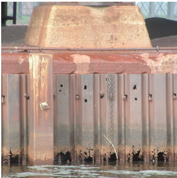
Widespread corrosion at Hancock, Michigan, (above) and Canadian National docks, Duluth, Minnesota (below)
